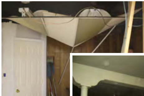
Left: WM Carl Lee attacks the old walls. Above: The old drop ceiling comes down. Left: The ceiling beam and column is uncovered.
